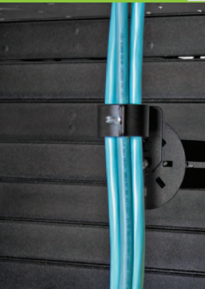
Rack-Mount Universal Clamp Kit Installed
